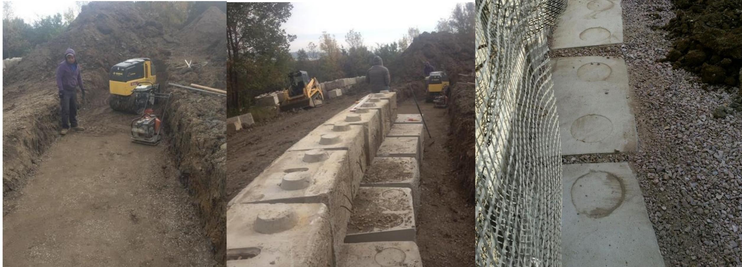
Compact your 6-8" base of gravel or crushed concrete with a packer then you can start placing your base blocks. If you are going over 8' high I would recommend using our 4400# base blocks. They will give you an excellent foundation for placing the rest of the blocks on. You may have to use more than one row of base blocks depending on your soil and height of your wall. You can also use geogrid to reinforce your wall or use a combination of both depending on your situation.
